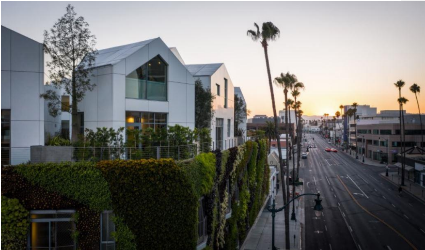
Green Wall example in Beverly Hills. Source: Darren Bradley
